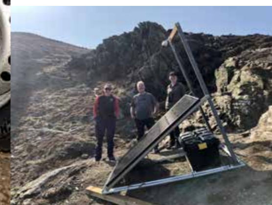
Volunteer, Kate Silverthorne with Aron Sapsford and Lara Howe, installing the Manx shearwater equipment on the Calf
